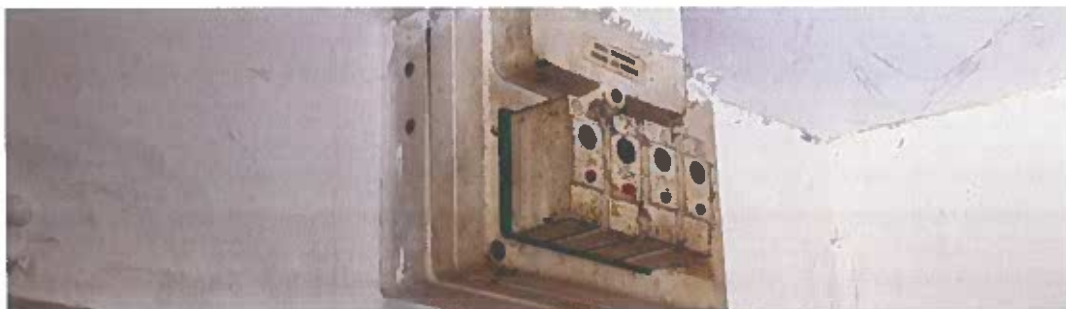
Nonstandard fuse board.
