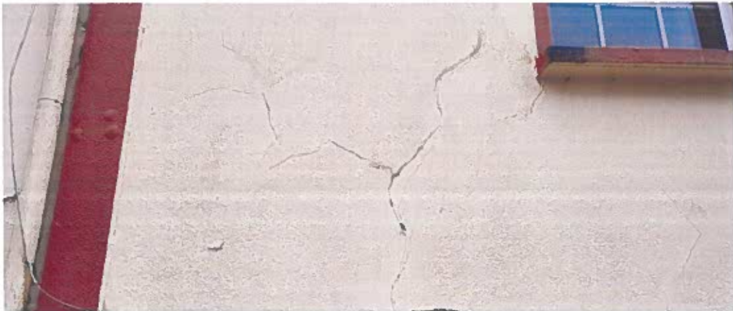
Cracks in plaster
