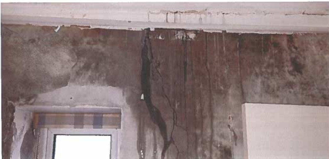
Roof leaking in bathroom.
