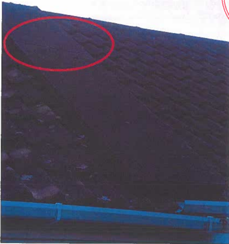
Image 4: Cracked Roof Barge
