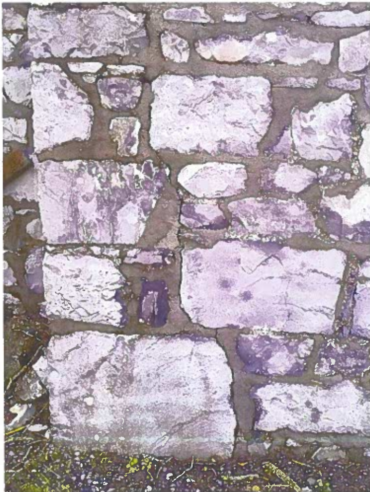
Structural crack which measures approximately 3-4mm in width. This property is derelict.
