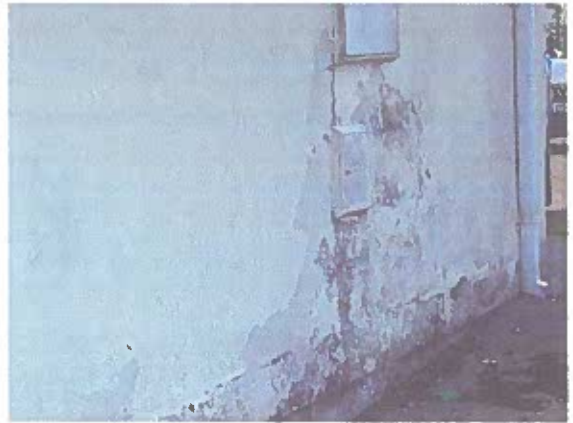
Figure 12: Cracks to be filled and dwelling painted
