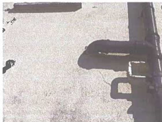
Figure 04: Pipework to be replaced
