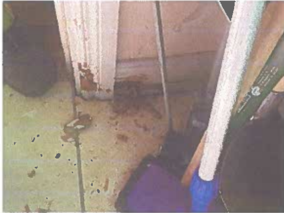
Figure 05: Dry rot noted to ground floor
