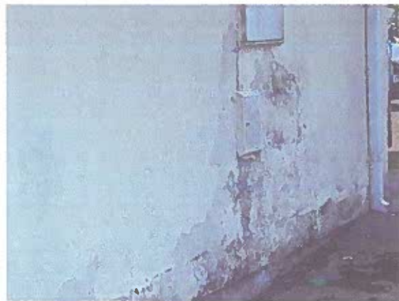
Figure 02: External crack to be filled and house painted
