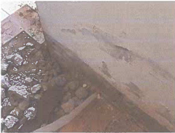
Figure 11: Floors to be removed, insulated and re-laid
