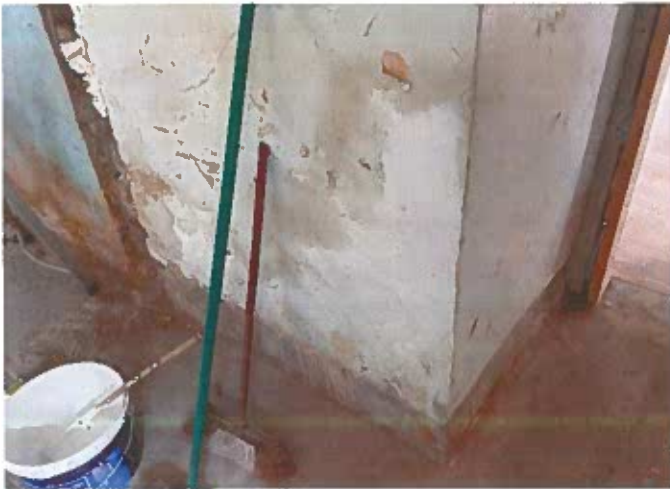
Photos 08b & 08c. There is evidence of damp on the base of the chimney wall, on each side.
