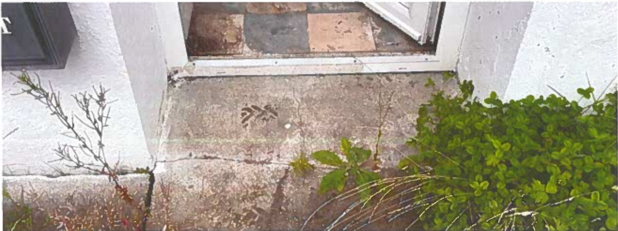
Photo 12. The ground level around the cottage is at the same level as the F.F.L. of the cottage.
