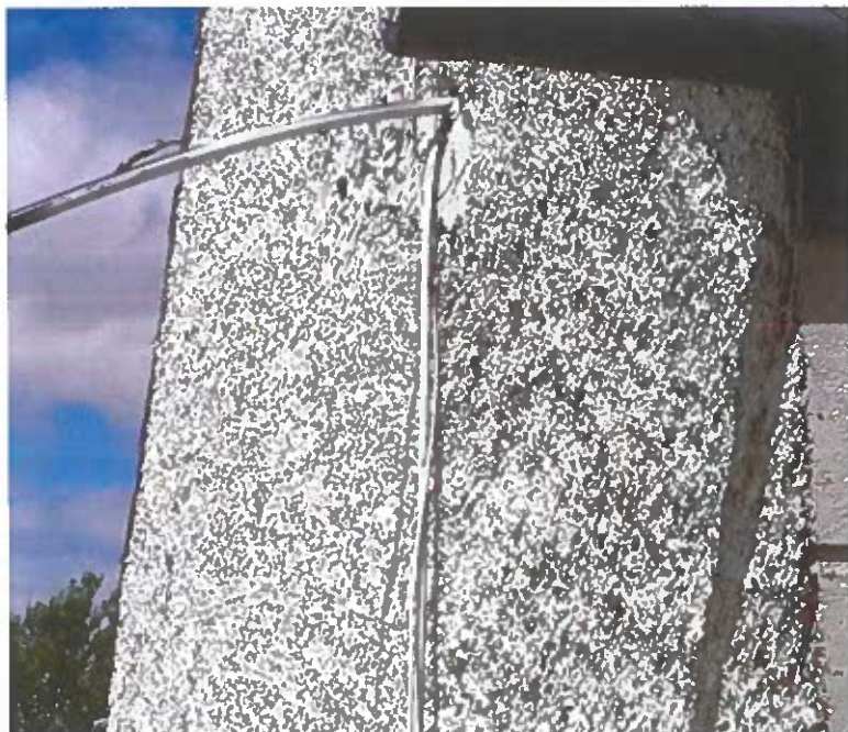
Photo 06. PVC gutter and downpipe. Note the rotten timber fascia board.
