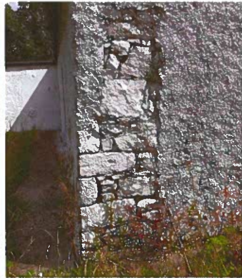
Photo 07b. The condition of the North\East external gable wall is in poor condition. Stones have fallen out in a several places and the stonework is poorly pointed. Photo 07c. Part of the South\West external gable wall is unrendered.
