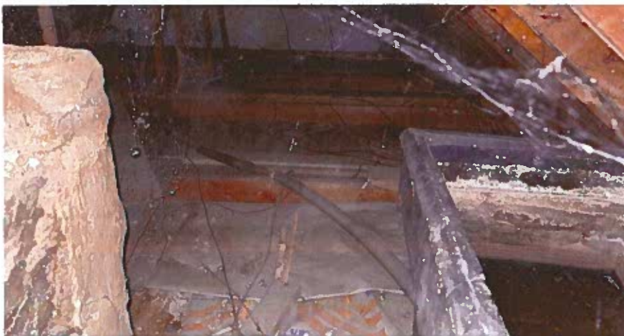
Photo 11a. There is no quilt insulation in the attic. The access hatches are not insulated or draughtproofed.
