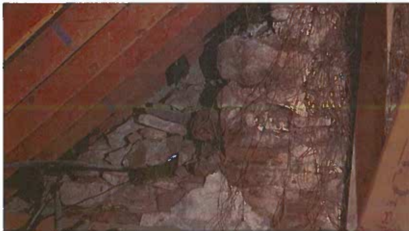
Photo 07d. The south\west gable wall in the attic is in a dilapidated condition.
