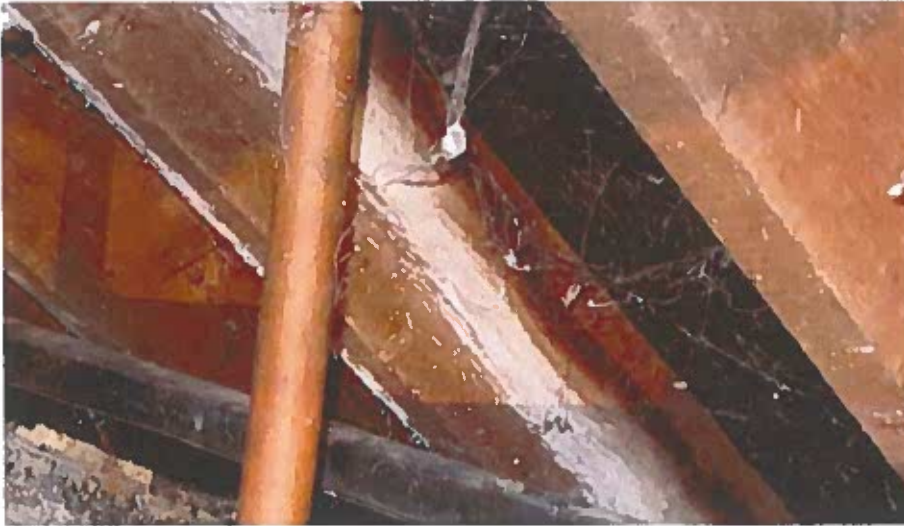
Photo 11b. The roof is a replacement roof as there is a black nonbreathable felt under the slates. Note the white mould staining on the rafters formed largely due to lack of ventilation.
