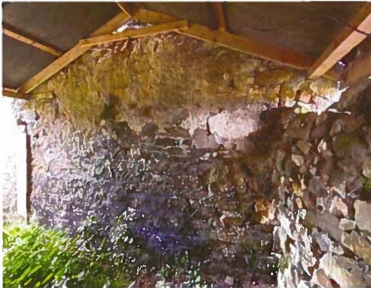
Photo 07b. The condition of the North\East external gable wall is in poor condition. Stones have fallen out in a several places and the stonework is poorly pointed. Photo 07c. Part of the South\West external gable wall is unrendered.
