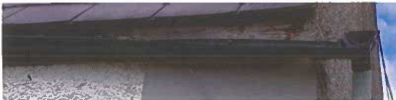
Photo 06. PVC gutter and downpipe. Note the rotten timber fascia board.
