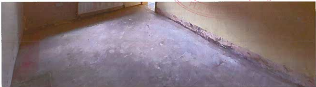
Photo 10. The original cottage floors were removed in the past and replaced with concrete floors. It is not possible to know whether insulation was used in the floor buildup or not, but it is unlikely. An impervious floor such as this prevents moisture from evaporating through the floor. The moisture therefore can tend to rise by capillary action up the stone rubble walls, leading to rising damp.
