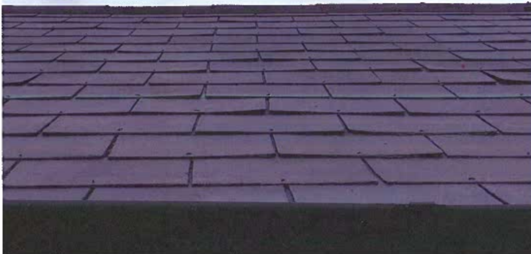
Photo 04a. Front roof plane. Note the curling up of the manmade slates.
