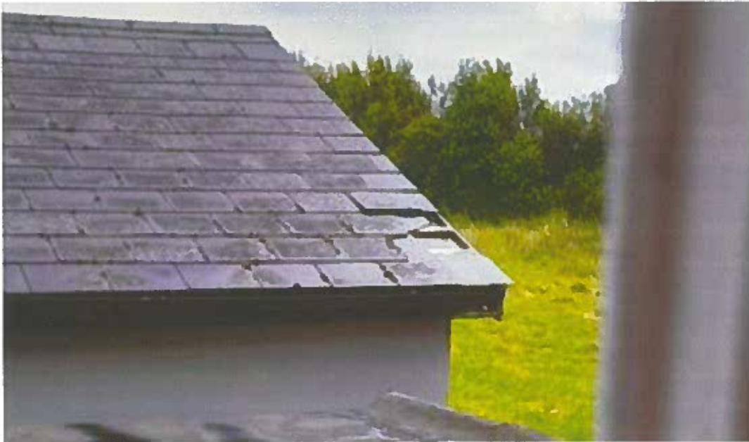
Photo 3 - Slipped/damaged slates to hipped roof
