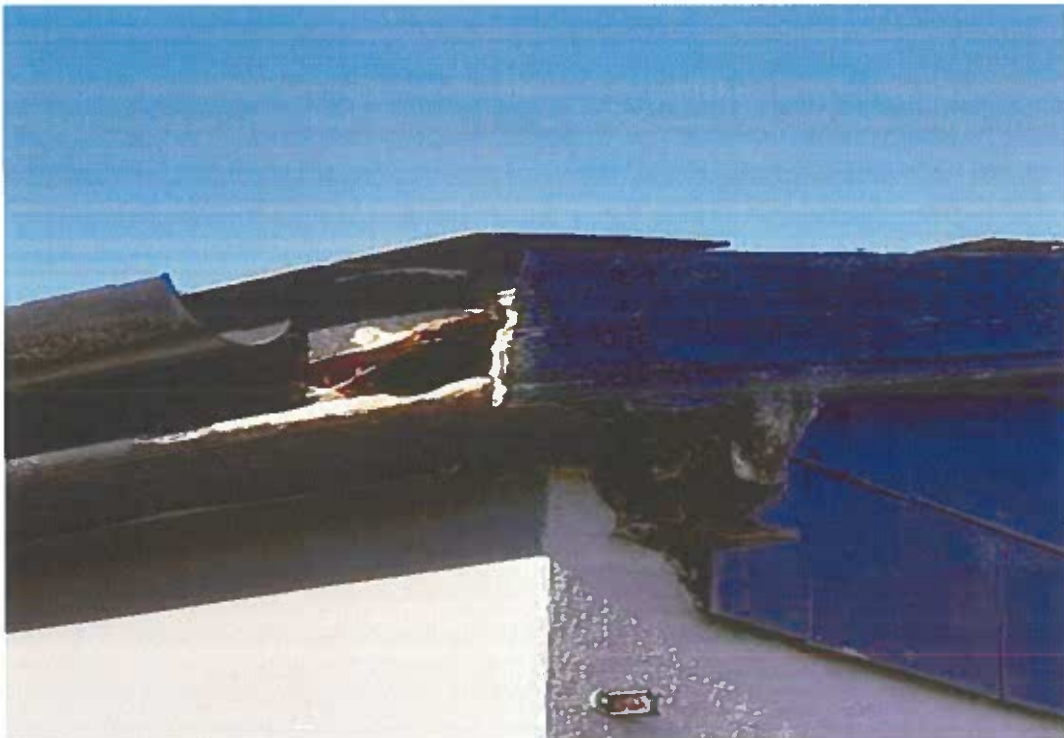
Photo 4 - Condition of timber fascia and soffit
