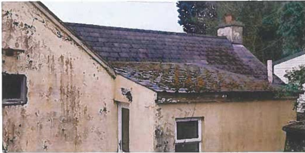
Existing flat roof extension with pitch of 10 degrees
