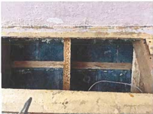
Photo 12. Roof timbers with no felt.
