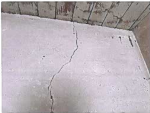
Photo 3. Hairline crack on wall.
