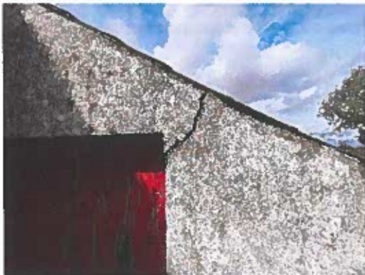
Photo 19. Crack on wall.
