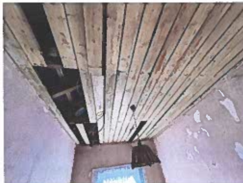
Photo 11. Ceiling boards missing.
