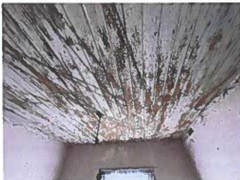
Photo 10. Damp spot on ceiling.
