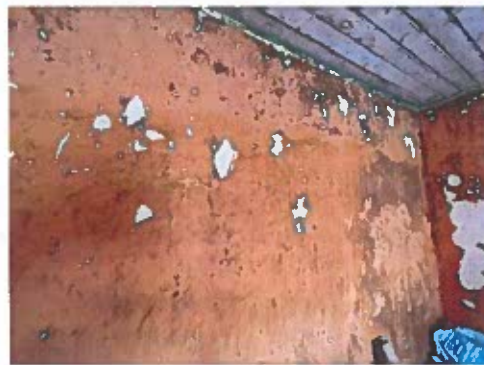
Photo 4. Damp stains on walls.
