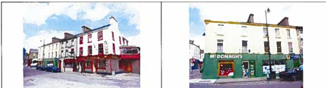
East side of Bridge Street. The traditional finish on the buildings in Boyle is a painted lime render, often ruled and lined and sometimes having quoins. This should be repaired and maintained and regularly painted as at McDonagh's.
