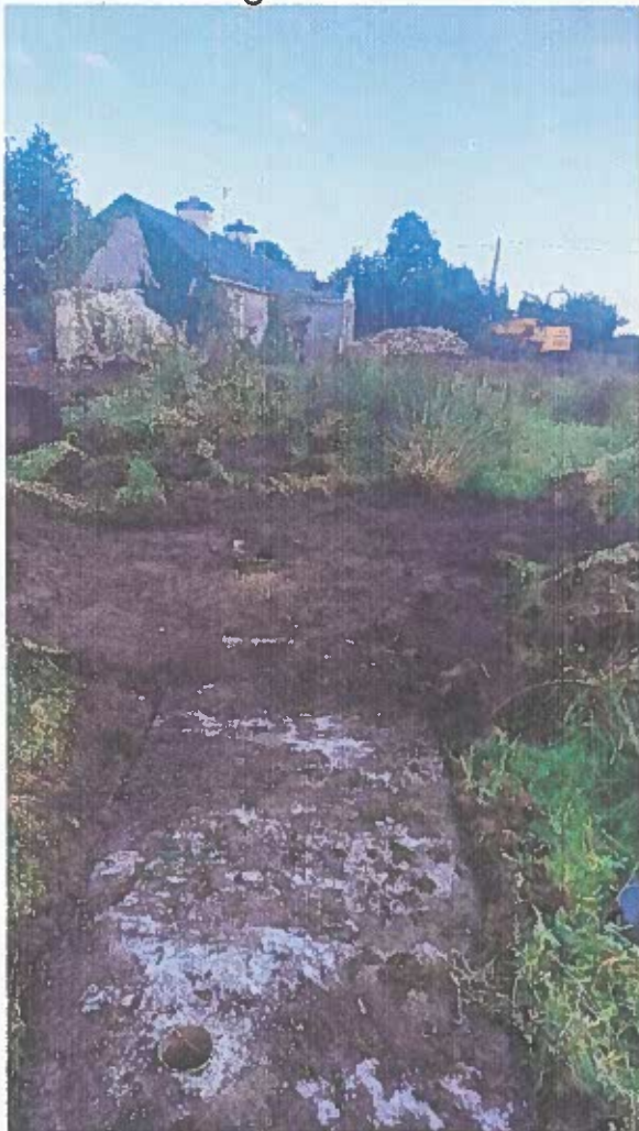
Existing 6m3 capacity 2 chamber fully functional Septic tank and soakpit onsite, house in background
