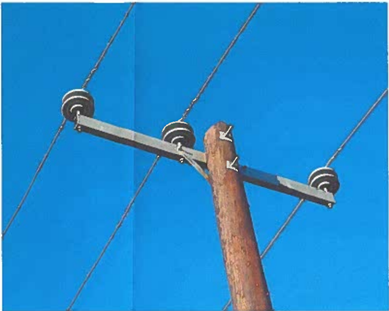
VIEW OF INTERMEDIATE POLE HEAD
