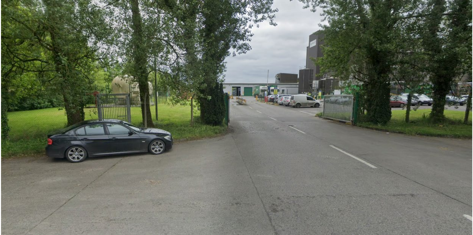
Figure 1 overall site entrance
