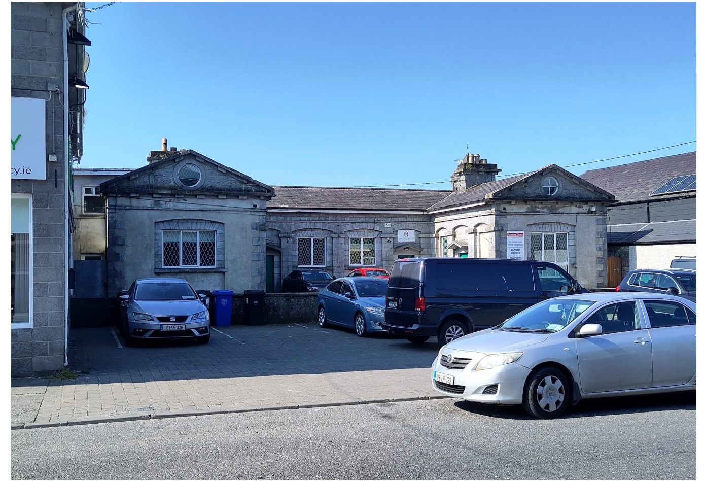
Current condition of the Old School House
