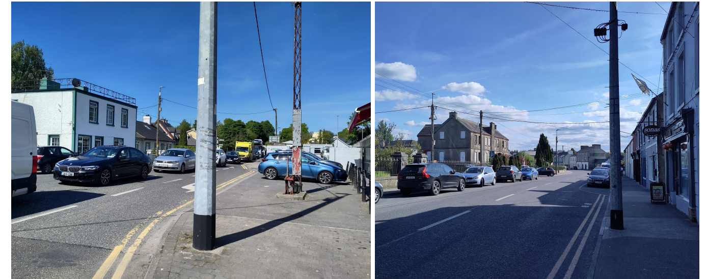
Current appearance of Gateways into Castlerea town centre
