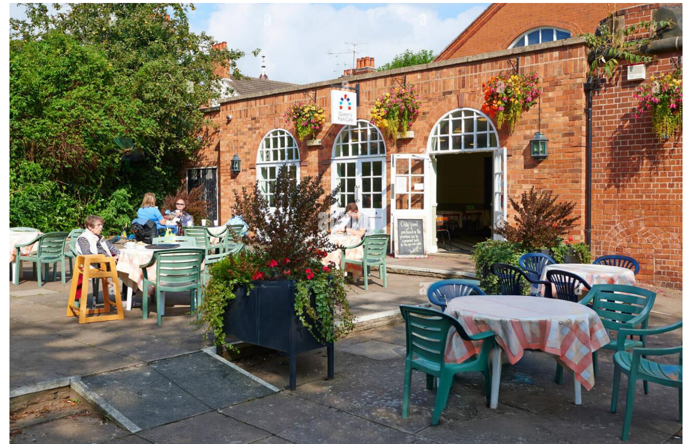
Restoration of former Gatehouse into a café
