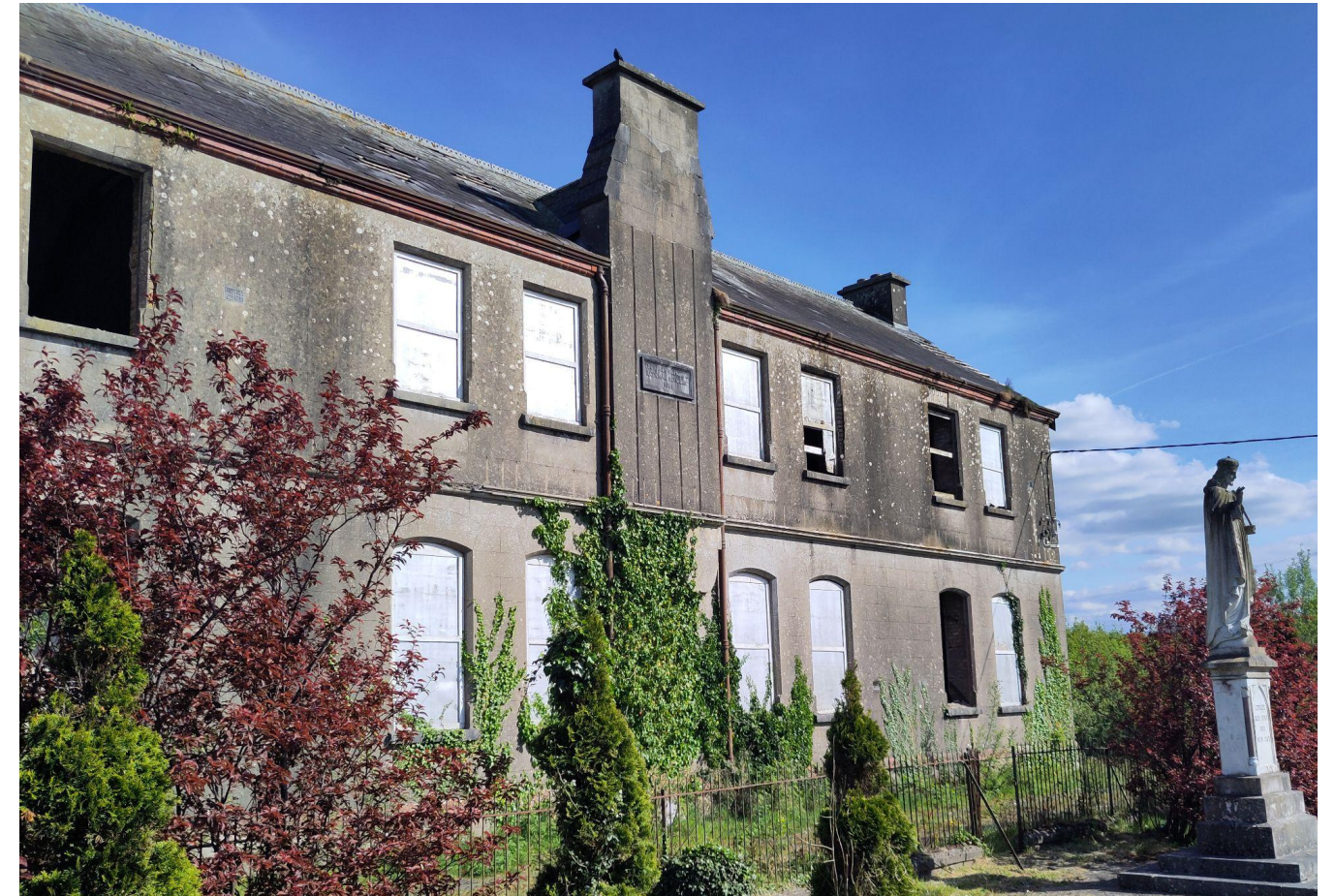
Current condition of the Hanly Hall
