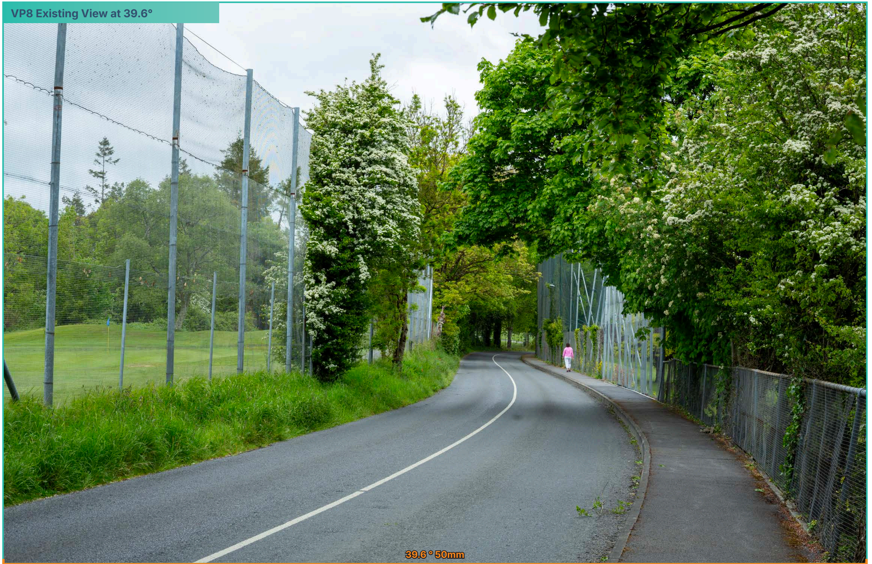
Viewpoint 08: View from the L2020 Local Road facing north, focused on the area of road widening along the site access route, with mature trees and golf-stop netting to be altered on either side of the road..
