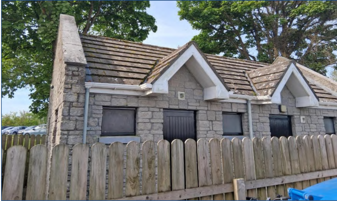
Plate 6-14. A representative photo of the toilets classed as Buildings and artificial surfaces (BL3) , which are proposed for demolition
