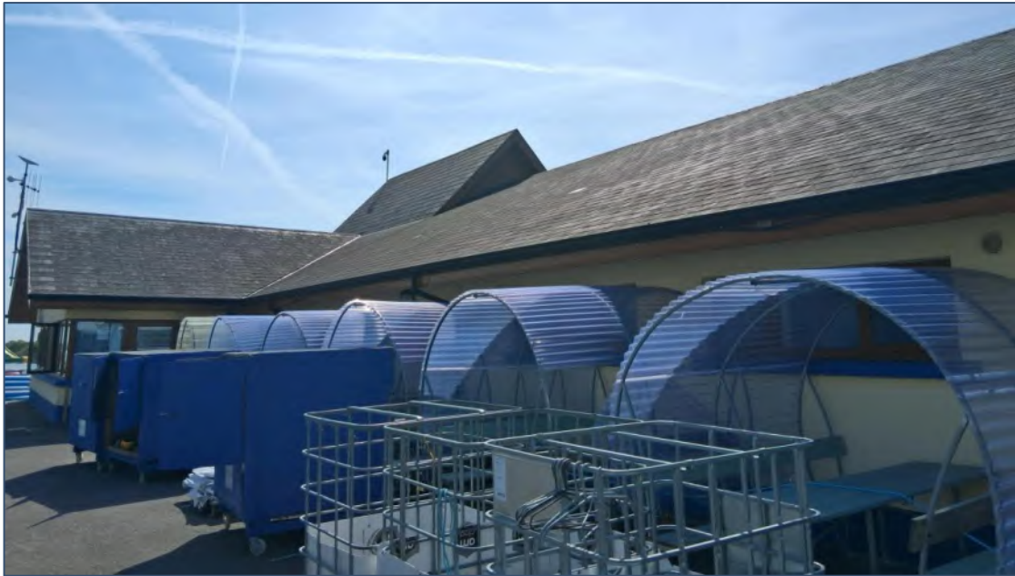
Plate 6-12. A representative photo of one of the Baysports buildings, classed as Buildings and artificial surfaces (BL3) , which is proposed for demolition.
