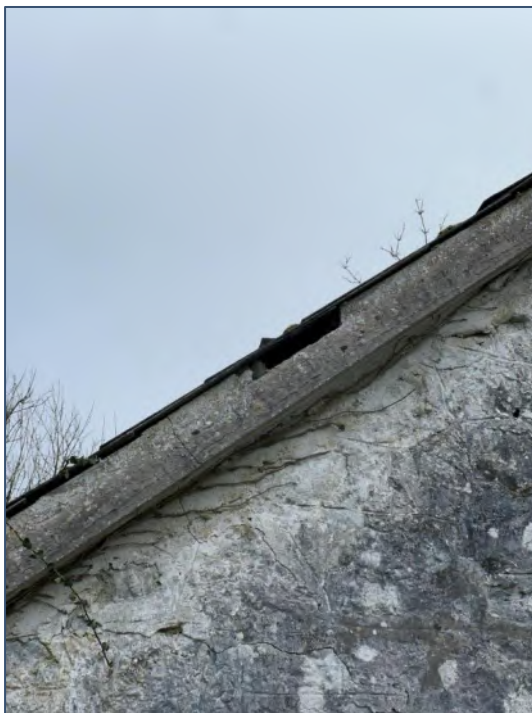
Plate 6-48. Representative images of gaps along the eaves of the southwestern end of the derelict railway building
