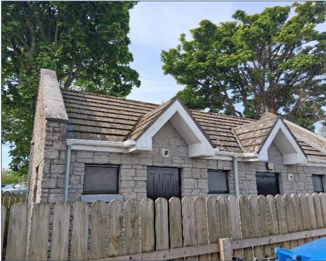
Plate 6-41. A representative image of the Public Toilet Block Building
