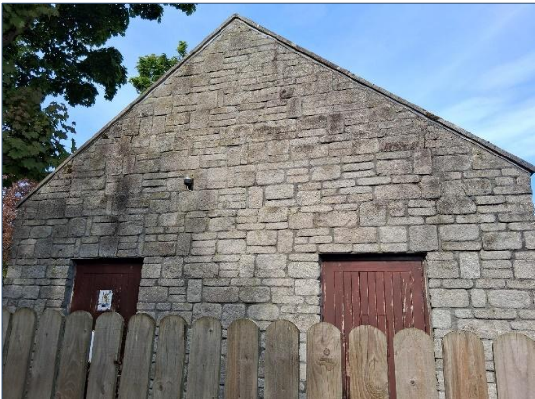
Plate 6-42. A representative image of the end of the Public Toilet Block Building
