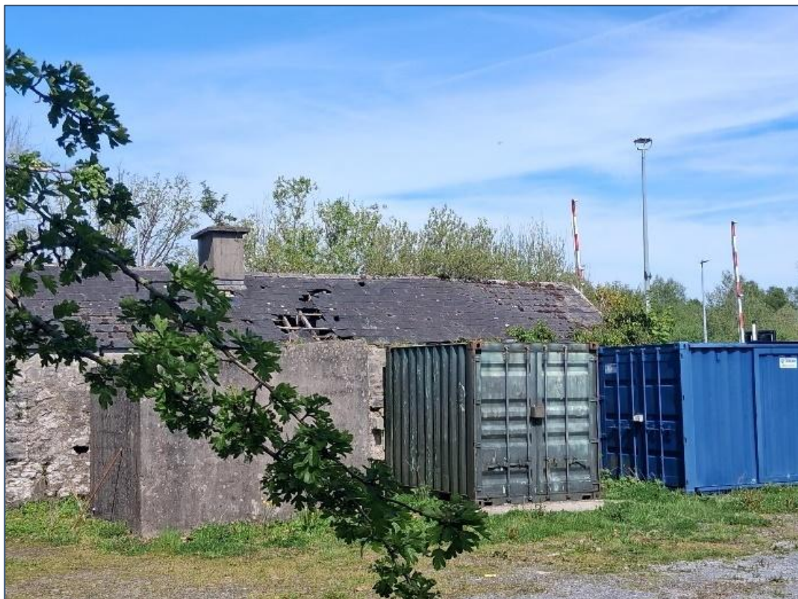
Plate 6-46. A representative image of the back of the derelict railway building, located outside of the Proposed Development Site.
