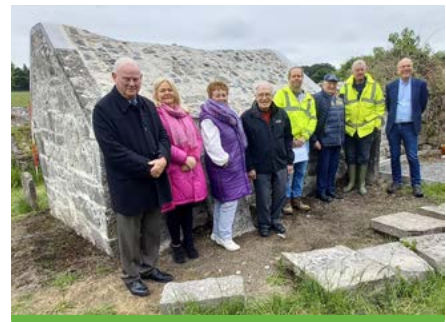
Viewing the completed conservation works to the Owen O'Connor mausoleum in Ballintubber, Piers O'Connor Nash; Eileen Kenny, Betty and Pat Garvey from Ballintubber Tidy Towns & Heritage and Fr. Pat O'Toole along with the project team - Niall Darroch, Stonemason, Eoin Halpin, Archaeologist and Michael O'Boyle, Conservation Architect.
