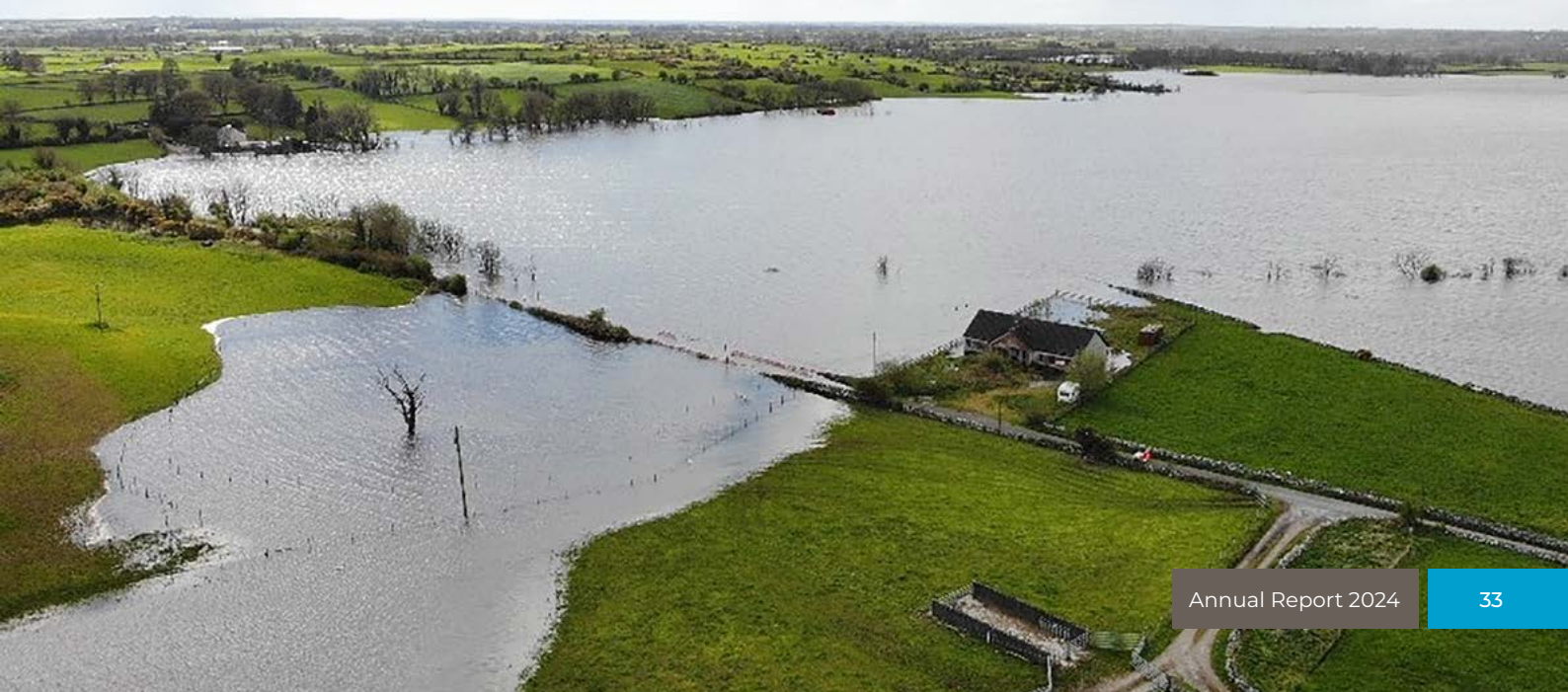
Lisphelim Local Road closed and under water.
