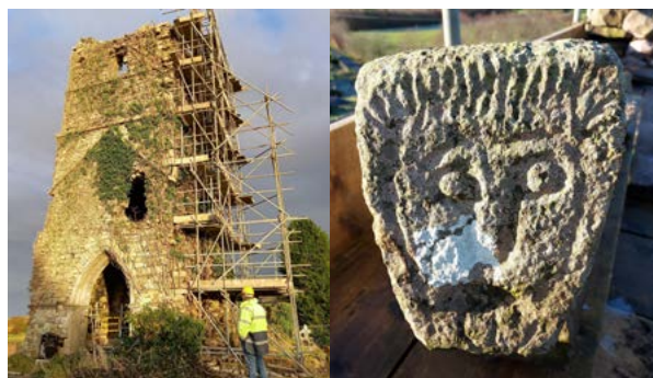
Phase 1 conservation works underway at Cloonshanville Abbey assisted by funding from the Community Monuments Fund.
