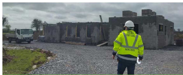
Building Control Inspection.
