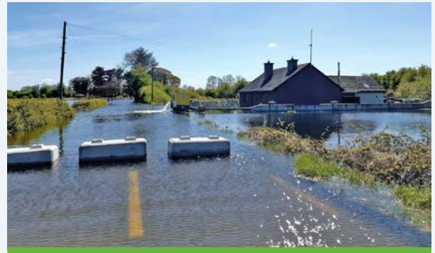
Regional Road under 750mm of water in Curraghboy.
