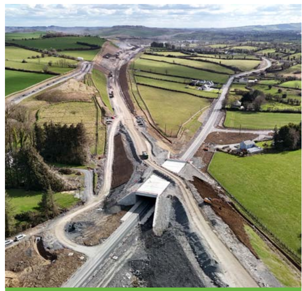
Ballaghaderreen to Scramoge Project.
