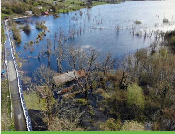
Aerial view of Ballagh Flood Defence.
