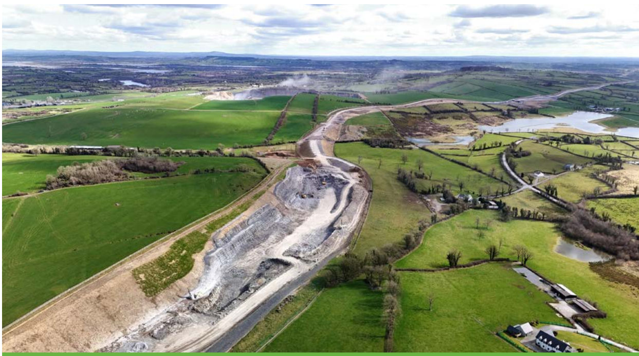
Ballaghaderreen to Scramoge Project.
