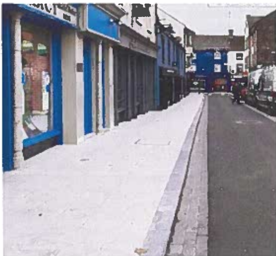
Ennis footpaths utilising Limestone kerbing and Granite Paving Slabs
