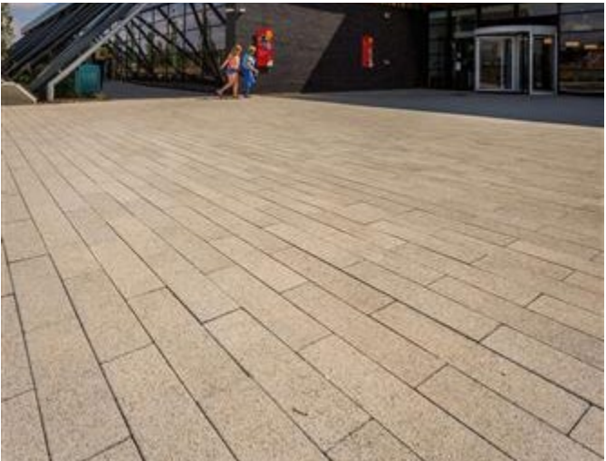
Example of concrete paving planks with exposed aggregate surface to the pedestrian footways
