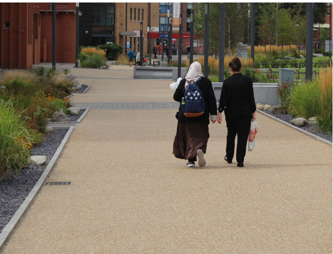
Example of insitu concrete surfacing with exposed aggregate surfacing to the Linear Park
