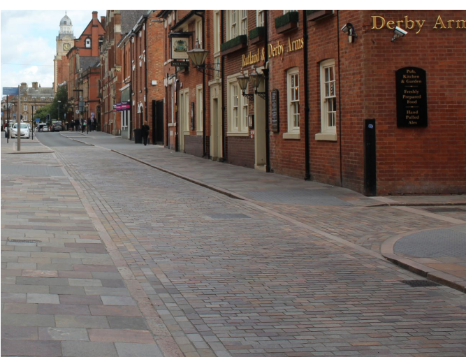
Example of natural stone surfacing upon the carriageways at key locations
