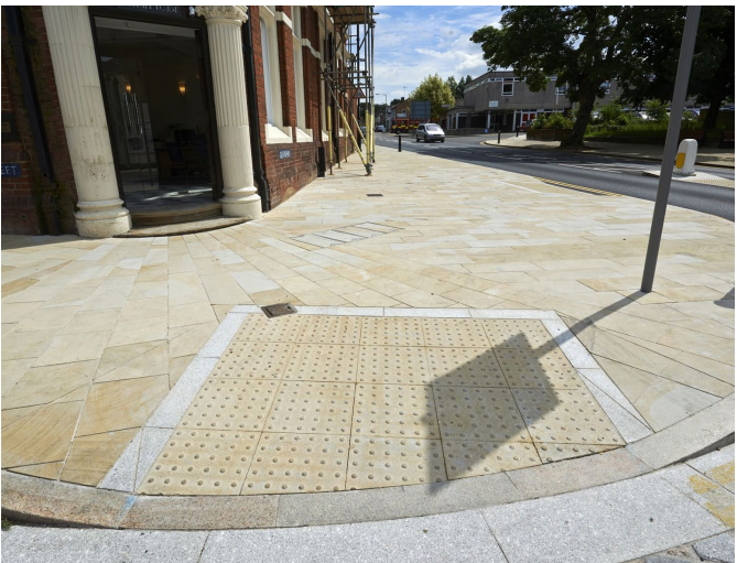
Example of blister paving demarcating crossing points throughout the scheme
