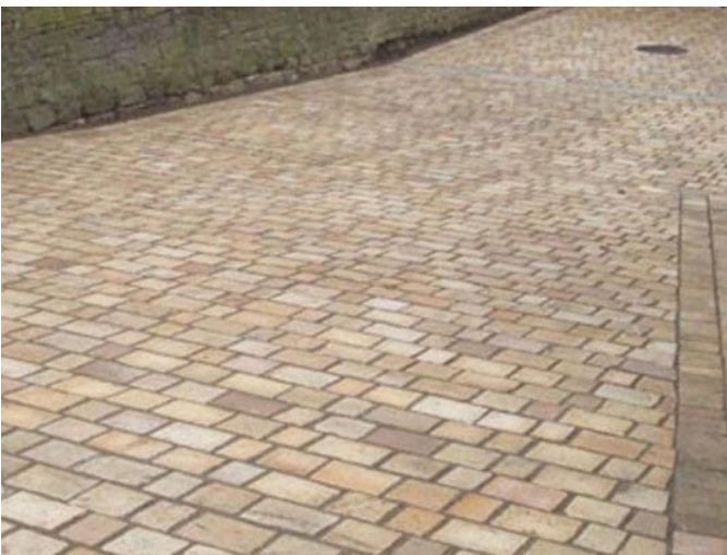
Example of high quality natural stone sett surfacing used at crossing points
