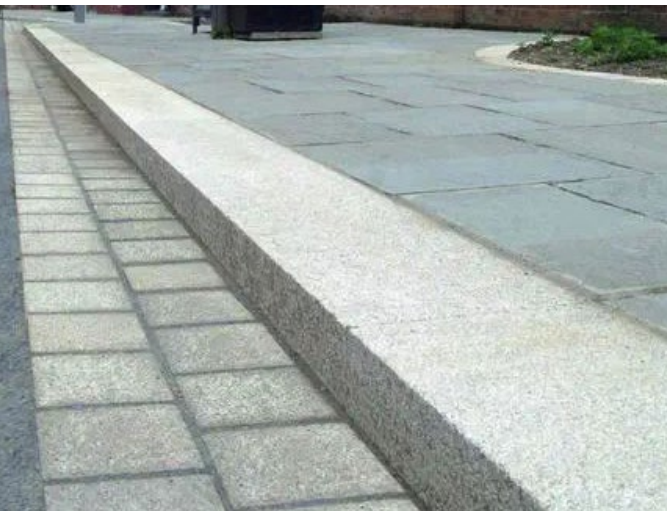
Example of wide natural stone kerbs used throughout the scheme
