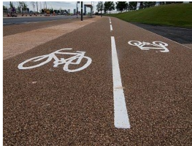
Example of coloured asphalt surfacing to the two-way cycleway
