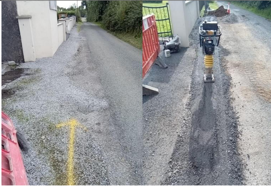
NBI backfilling / compacting trench as per purple book specifications
