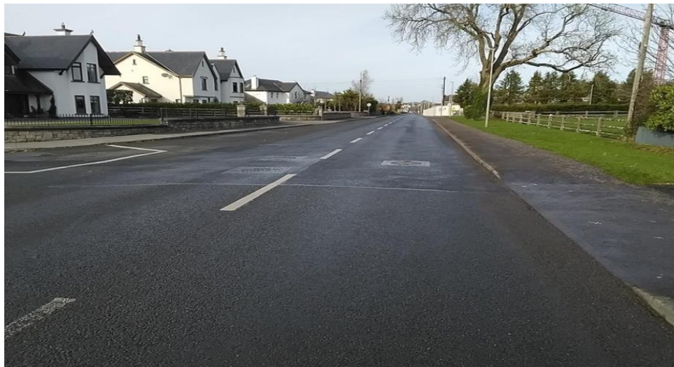
Image above of perfect full road width reinstatement inspected and accepted by Area Engineer
