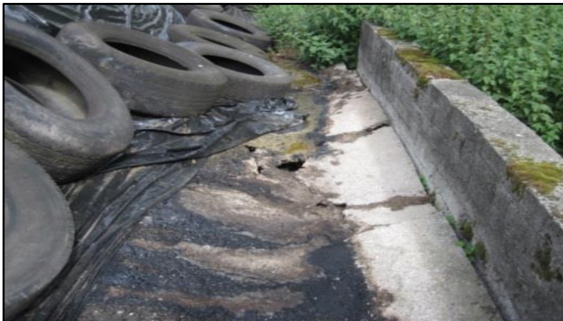
A cracked silage effluent channel allowing leakage (Photo: Andrew Holmes).
