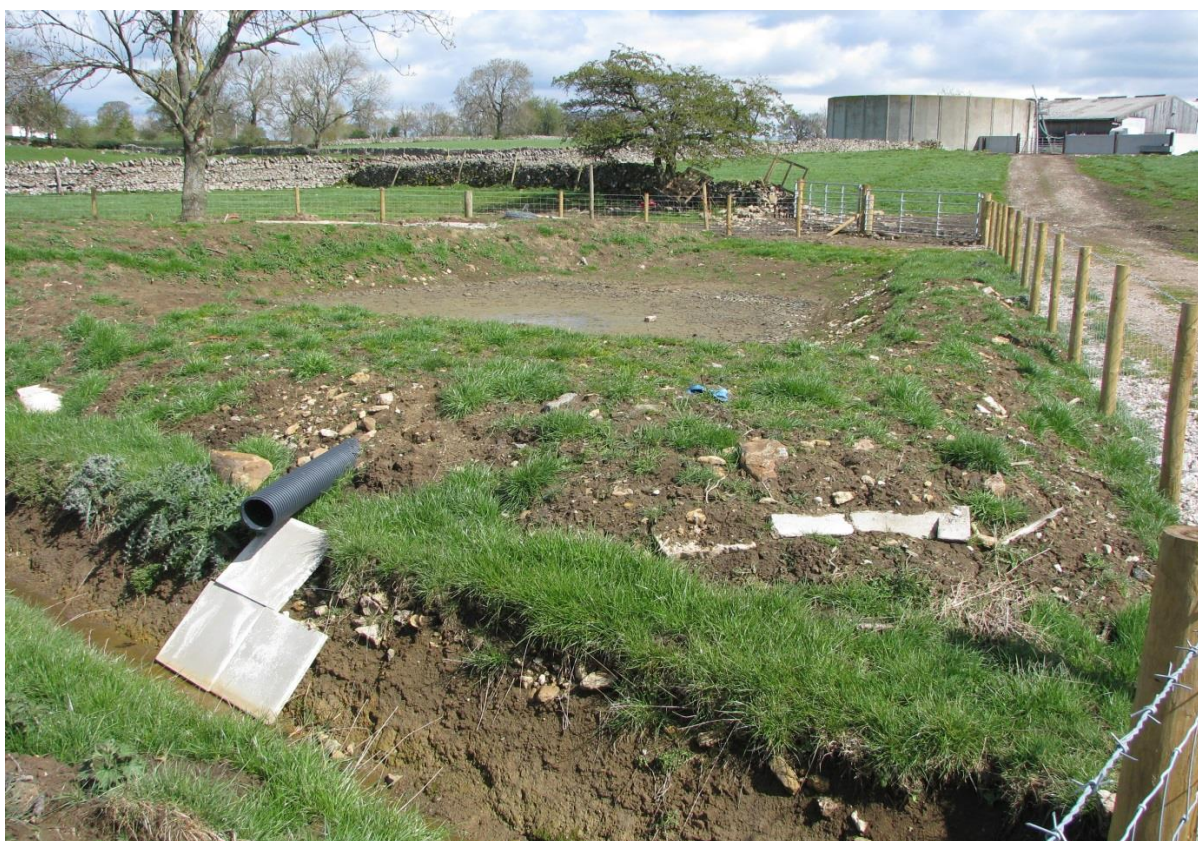
Runoff from the farm road is channelled into the sediment trap on the left (Photo: Donal Daly).
