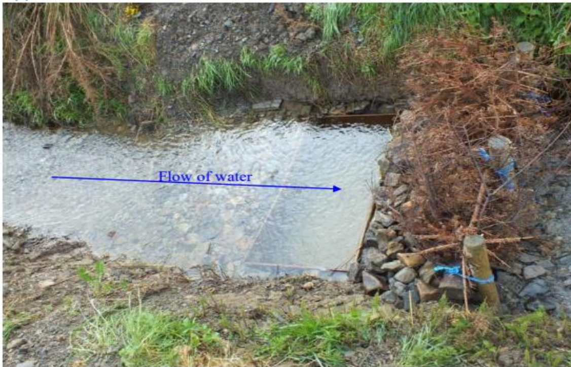
Figure 7 Silt trap installed in stream at Kilberriher
