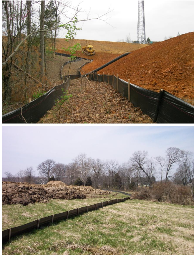
Plate 6.1 Typical Silt Fence Usage
