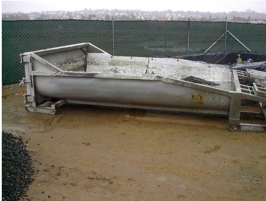
Plate 6.3 Typical Washout Facility
