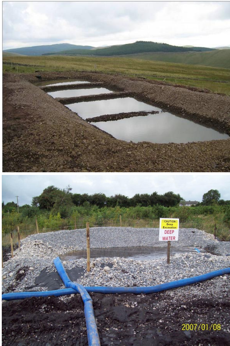
Plate 6.2 Typical Temporary Settlement Pond/Lagoon
