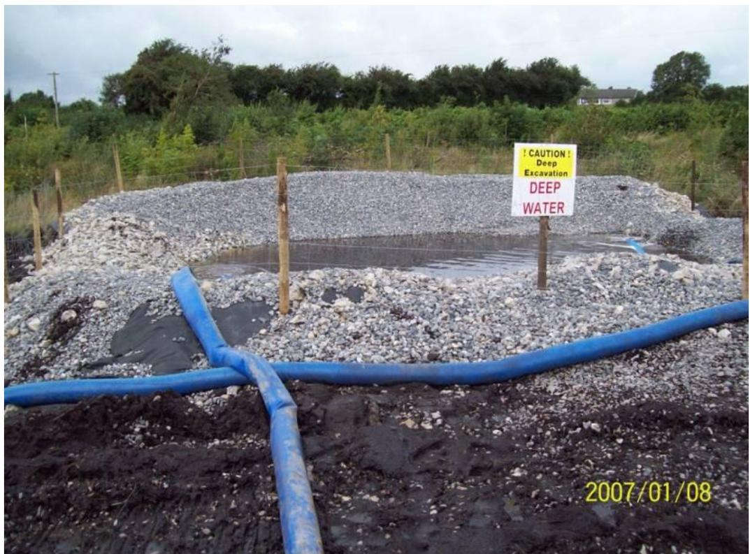
**Plate 6.2 Typical Temporary Settlement Pond/Lagoon**
