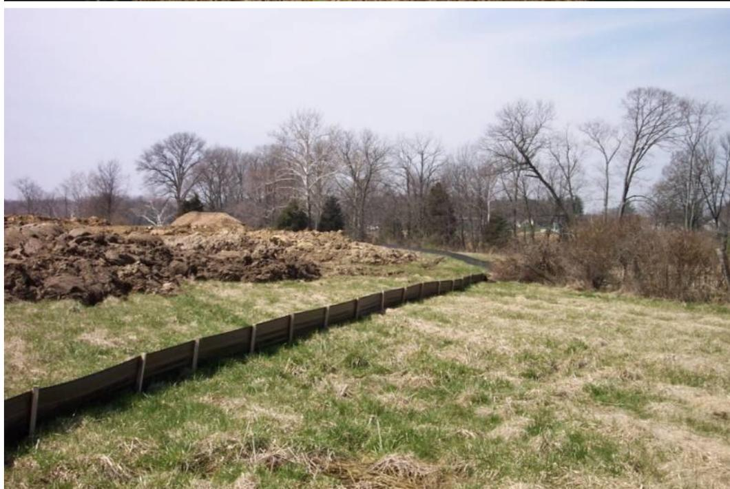
**Plate 6.1**                      **Typical Silt Fence Usage**
