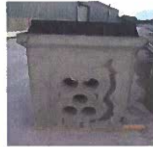
ESB Networks Approved Communication and Cable Screen Sectionalising Chamber
