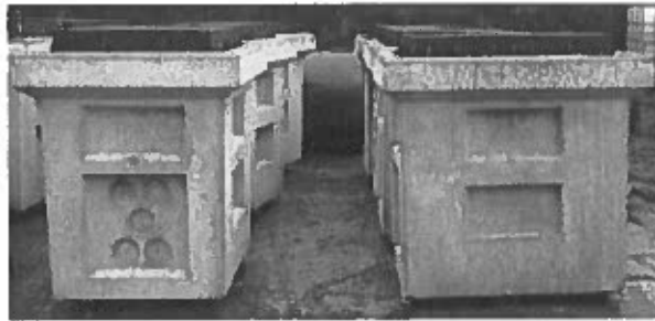
ESB Networks Approved Communication and Cable Screen Sectionalising Chamber
