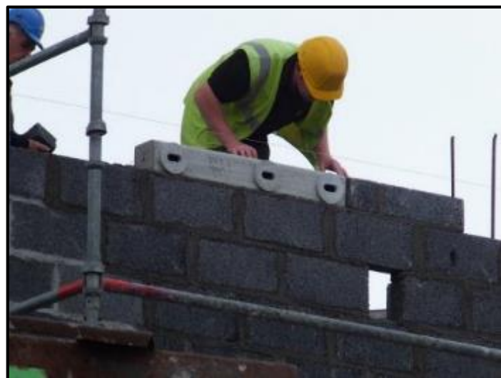
Figure 28: Installing Swift boxes as part of the fabric of the wall. Photo: Lynda Huxley
