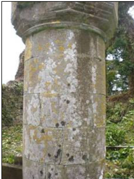
Figure 15: The cylindrical column has a number of vertical cracks in the stonework
