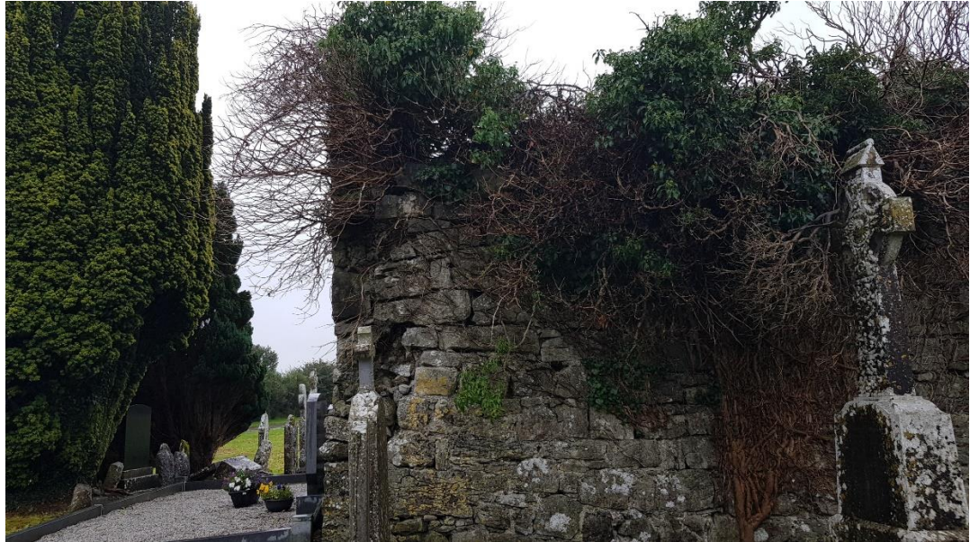
Fig. 9 Outward lean on east gable wall of Rahara Church. The dislodgement of stones at the corner appears to be linked to the movement in this wall.
