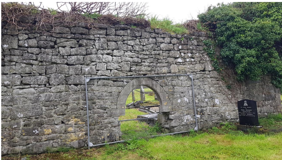
Fig. 4 Pointed arch door with cut limestone head on north exterior face of Rahara Church. The cut stone surround below this arch is missing.
