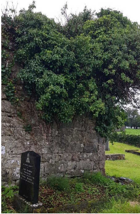
Fig. 12 Ivy growth on north wall (exterior face) at north-west corner
