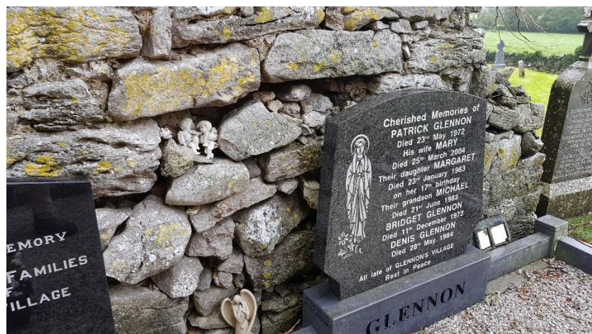
Fig. 11 Substantial gap at base of east gable (exterior face) that has been filled with loose stone.
