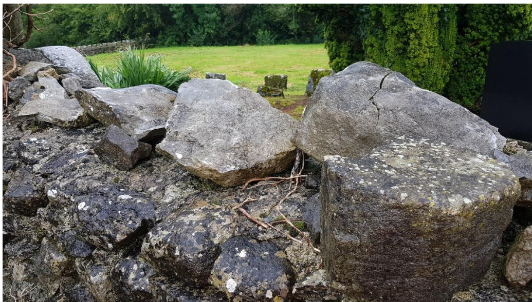
Fig. 16 Open gaps along the top of a truncated section of wall at the south gable. The individual stones at the top of the wall have been re-bedded in a cement mortar (during the twentieth century), which is significantly harder than the historic masonry and is contributing to instability in the wall.
