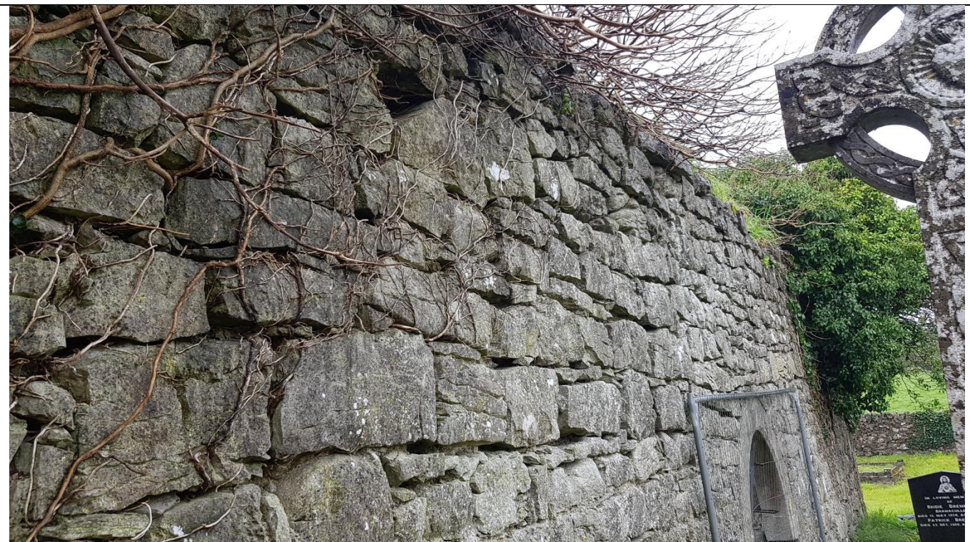
Fig. A4 Detail of stone rubble exterior face of north wall
