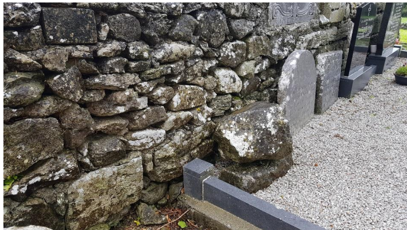
Fig. 10 Deep open joints in the stone rubble at the base of the east gable (exterior face)
