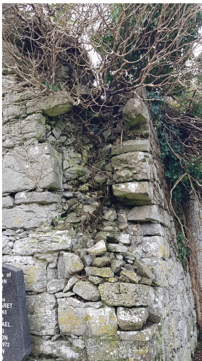
Fig. 8 Missing stone on north-east corner
