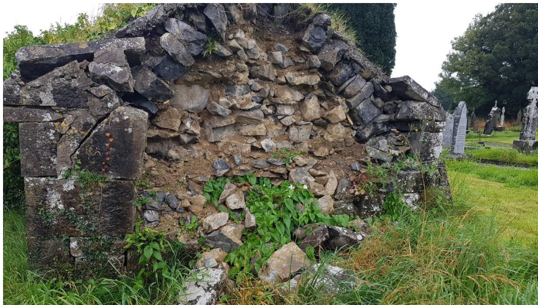
Fig. 8 Detail of collapsed east gable
