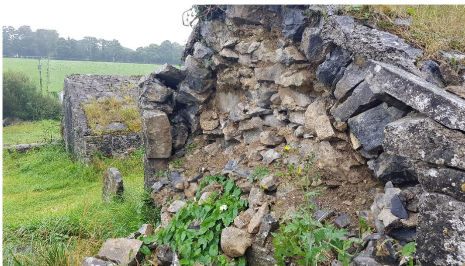
Fig. 5 Detail showing exposed inner vault construction at collapsed east gable of Owen O'Connor Mausoleum.
