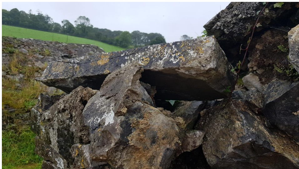
Fig. 10 Loose stones at edge of roof and east gable
