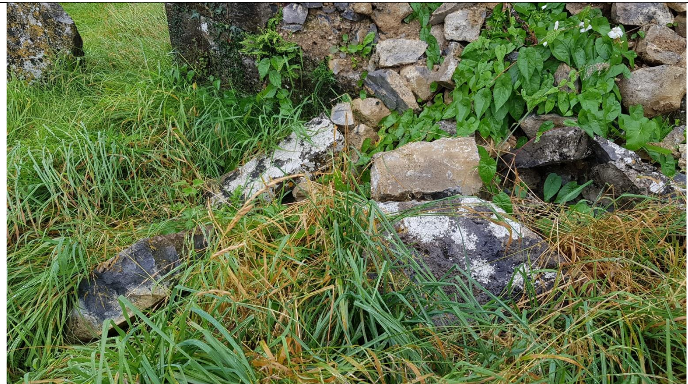
Fig. A3 Collapsed stone rubble at base of east gable
