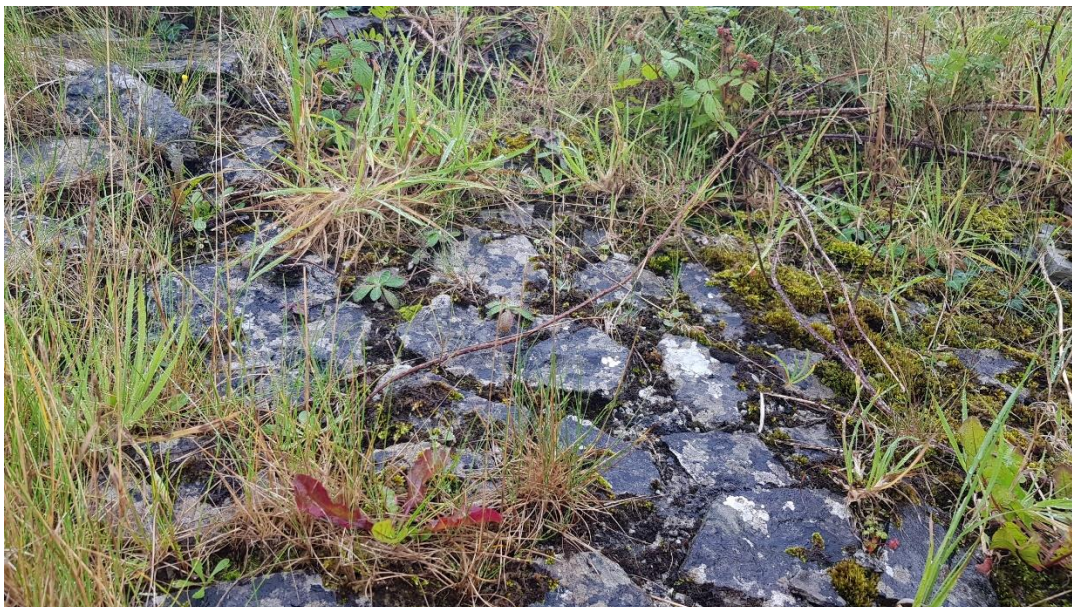
Fig. 6 Detail of flat limestone random slab finish to pitched roof of Owen O'Connor Mausoleum
