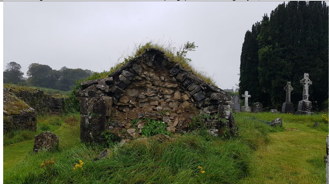
Fig. A2 Collapsed east gable of Owen O'Connell Mausoleum
