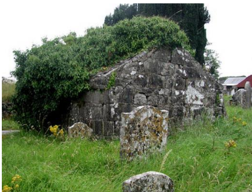
Fig. 3 Photograph of the east gable prior to the collapse of the stone facing, taken as part of the NIAH survey in August 2003 (NIAH ref. 31815002). The use of smaller stones under the barge is quite different to the cut stone lower down and suggests that the slope of the roof may have been changed.
