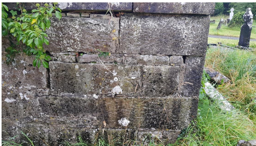
Fig. 11 Detail of squared limestone on south exterior face of Mausoleum, at corner with collapsed east gable.
