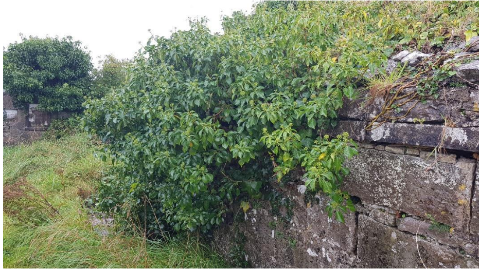
Fig. 12 Detail of squared limestone on south face of mausoleum, with heavy ivy growth on west gable
