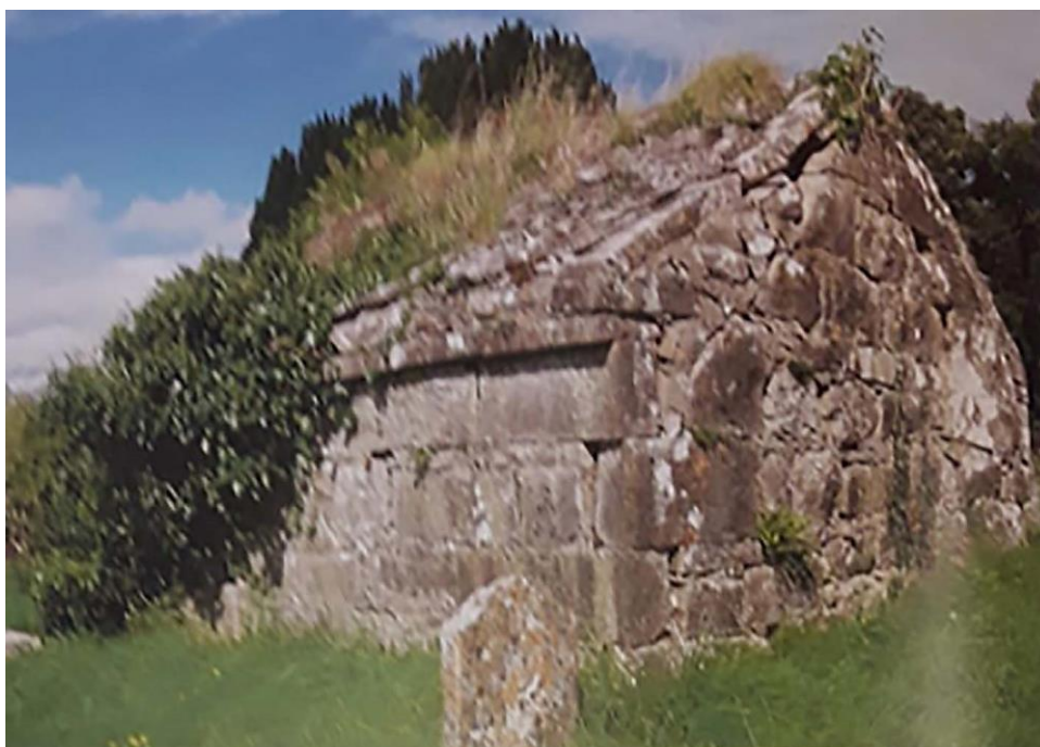
Fig. 7 Photograph of east gable shortly prior to its collapse, showing large gaps in the stone rubble under the south barge (2018, reproduced from Timoney, P. 182)
