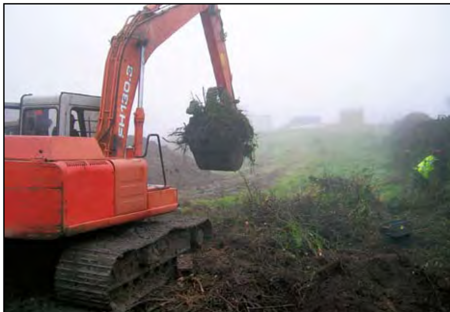
Photo 28: Stage 5 - Lifting the root ball
