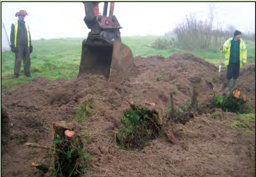
Photo 9: Backfilling of plants to stabilise them in position
