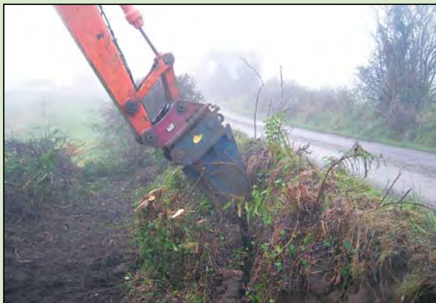
Photo 27: Stage 4 - Severing roots with cutting tool
