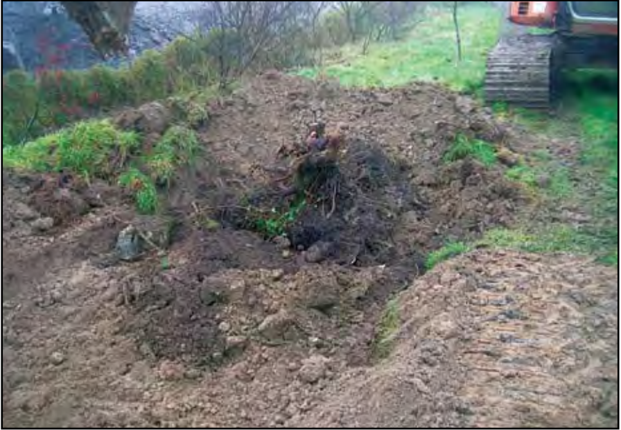
Photo 32: Stage 9 - Initial back-filling
