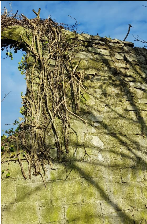
Fig. A37 Detail of external façade of apse (south side)
