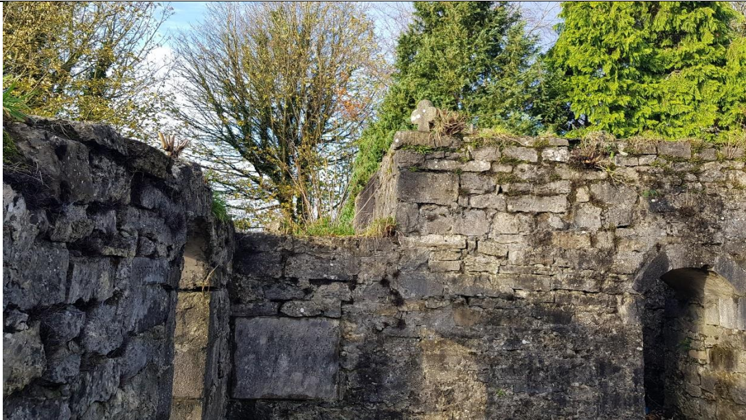
Fig. A19 West wall of nave (inner face) at junction with tower
