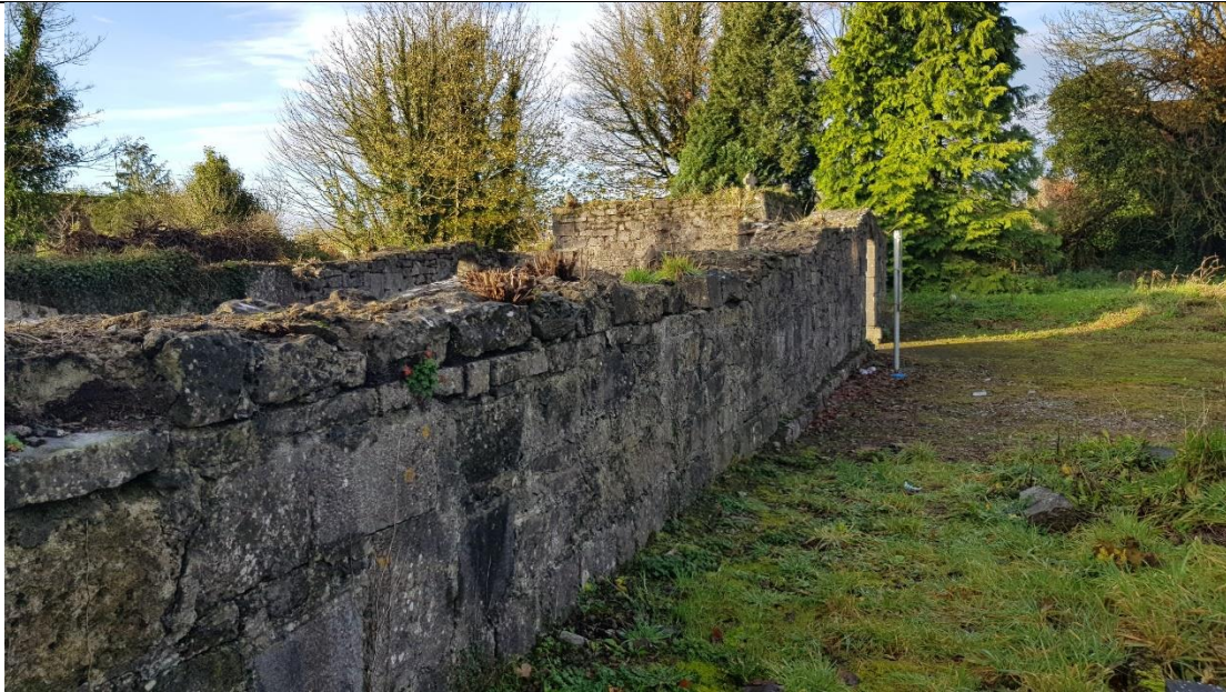
Fig. A32 North façade of nave, looking west towards tower
