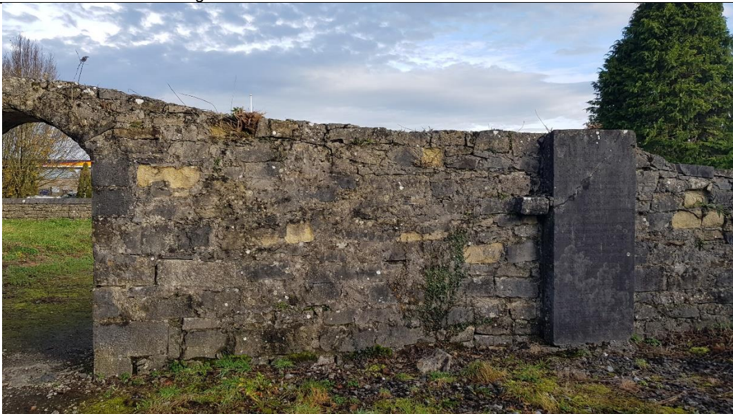
Fig A5 Internal face of north external wall to nave
