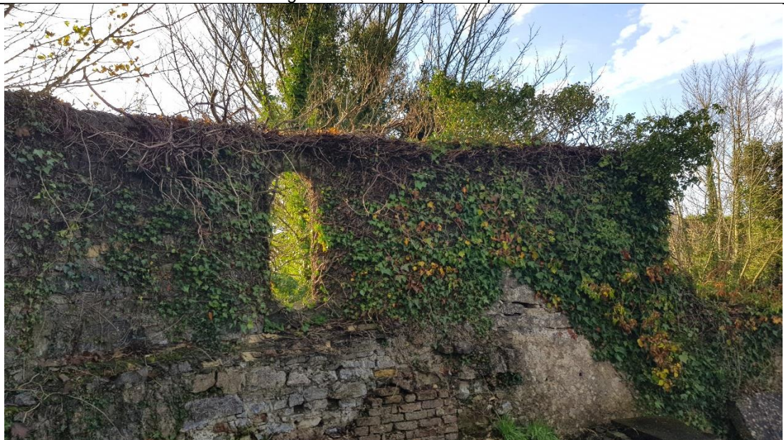
Fig. A15 Internal façade of apse
