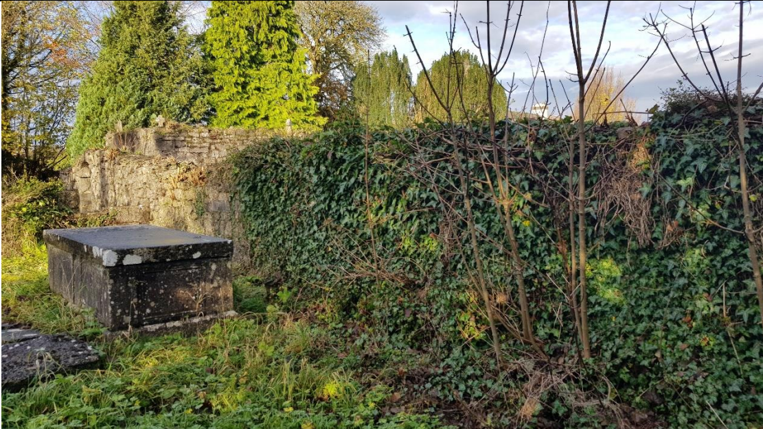
Fig. A40 South façade of nave, looking west towards chapter room; with mature saplings growing out of base of facade
