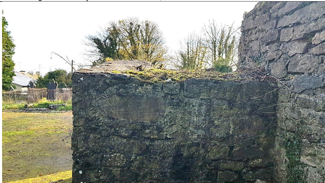
Fig. 51 West façade of nave, with tower on right
