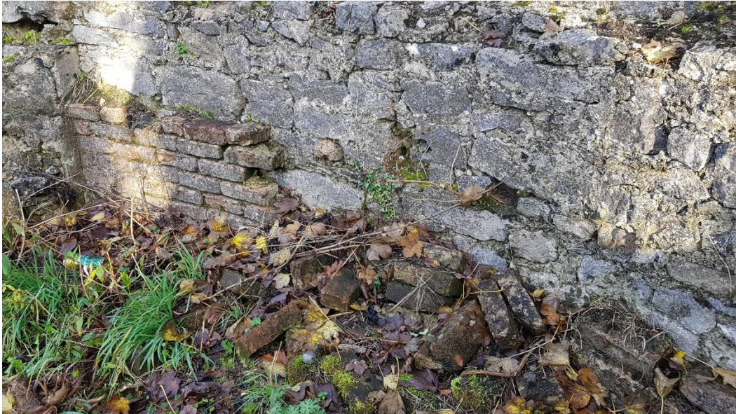
Fig. 8 Brick lining within apse
