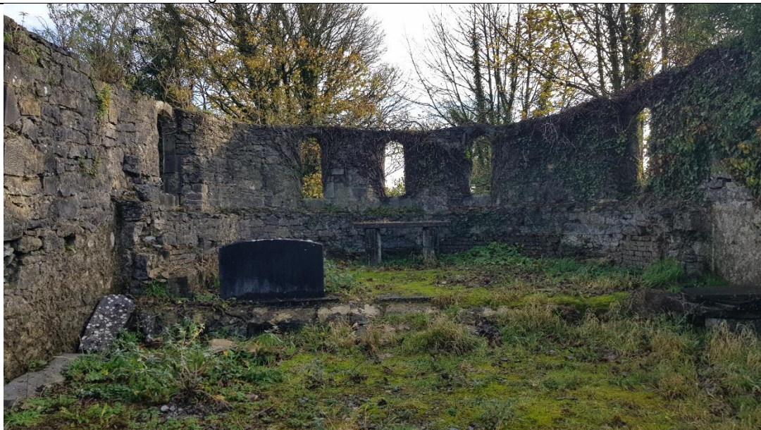
Fig. A9 Apse at east end of the nave
