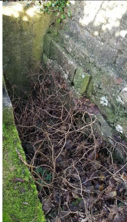
Fig. A38 External steps to crypt beneath nave
