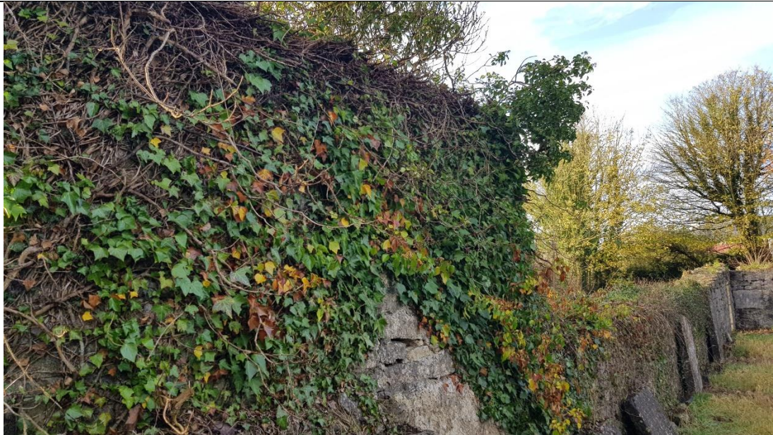
Fig. A16 South wall of nave, viewed from apse
