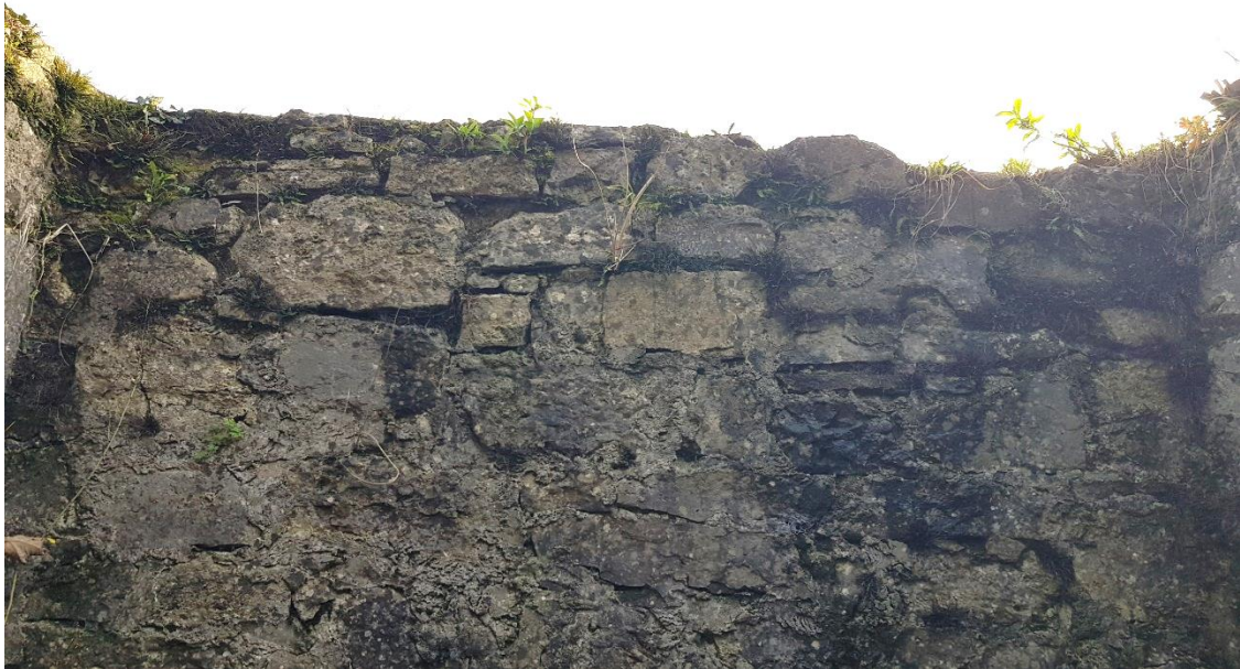
Fig. A24 Interior of rectangular tower, south wall
