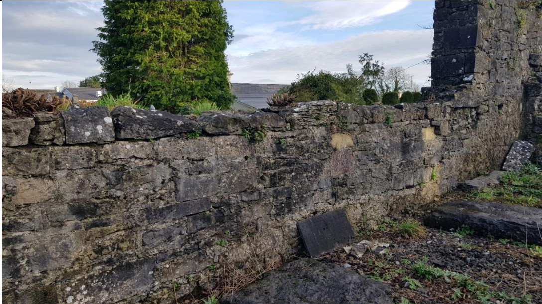
Fig. A8 Internal face of north external wall to nave
