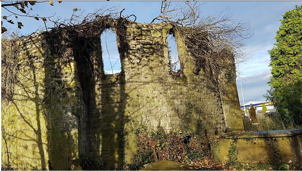
Fig. A36 External façade of apse
