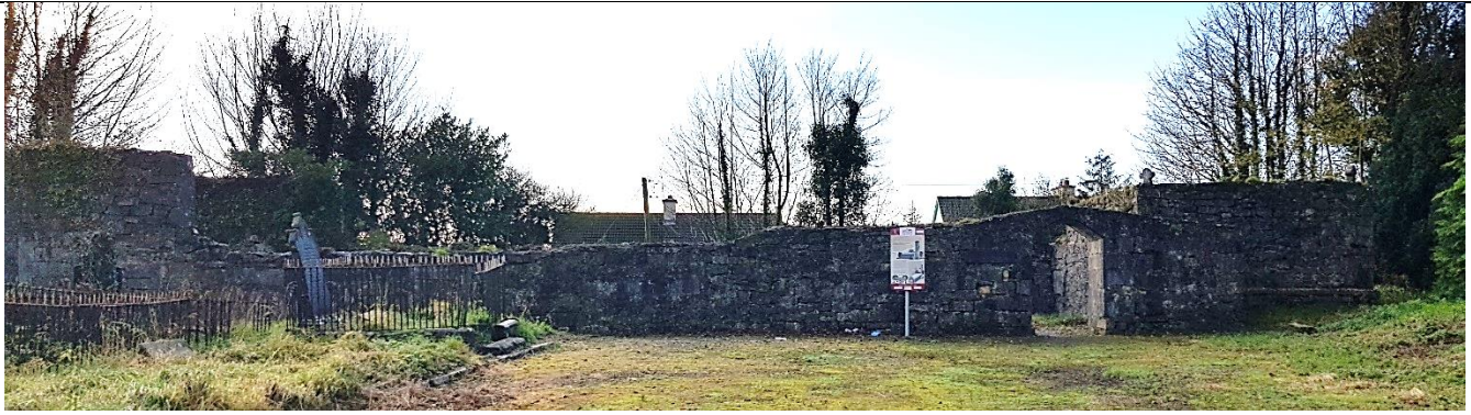
Fig. A1 North façade of St. Mary's Cathedral, viewed from Fair Green
