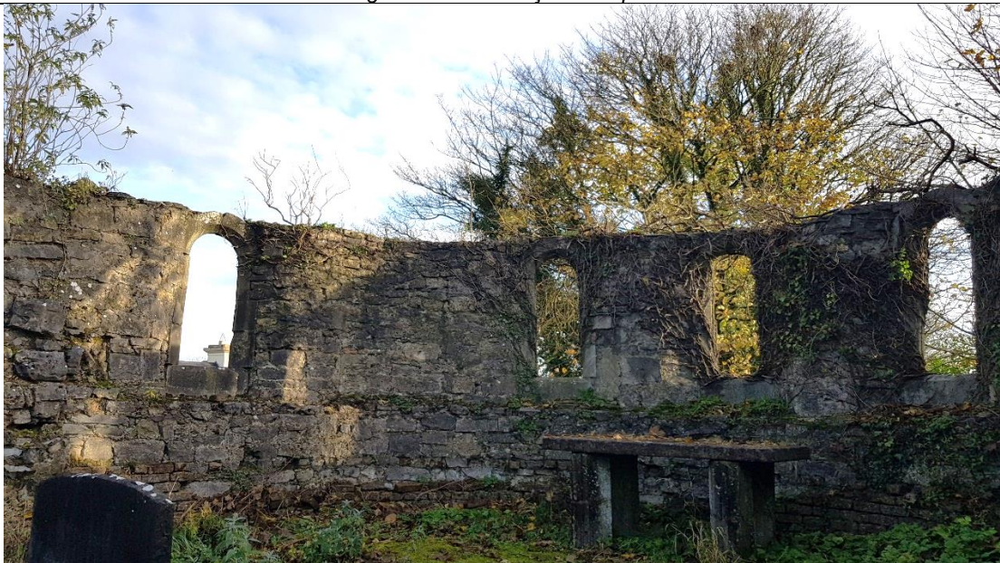
Fig. A14 Internal façade of apse
