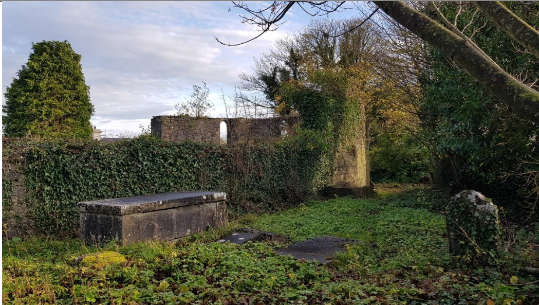
Fig. A42 South façade of nave, looking east towards apse
