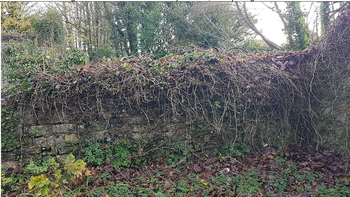
Fig. A31 Inner face of east wall of chapter room
