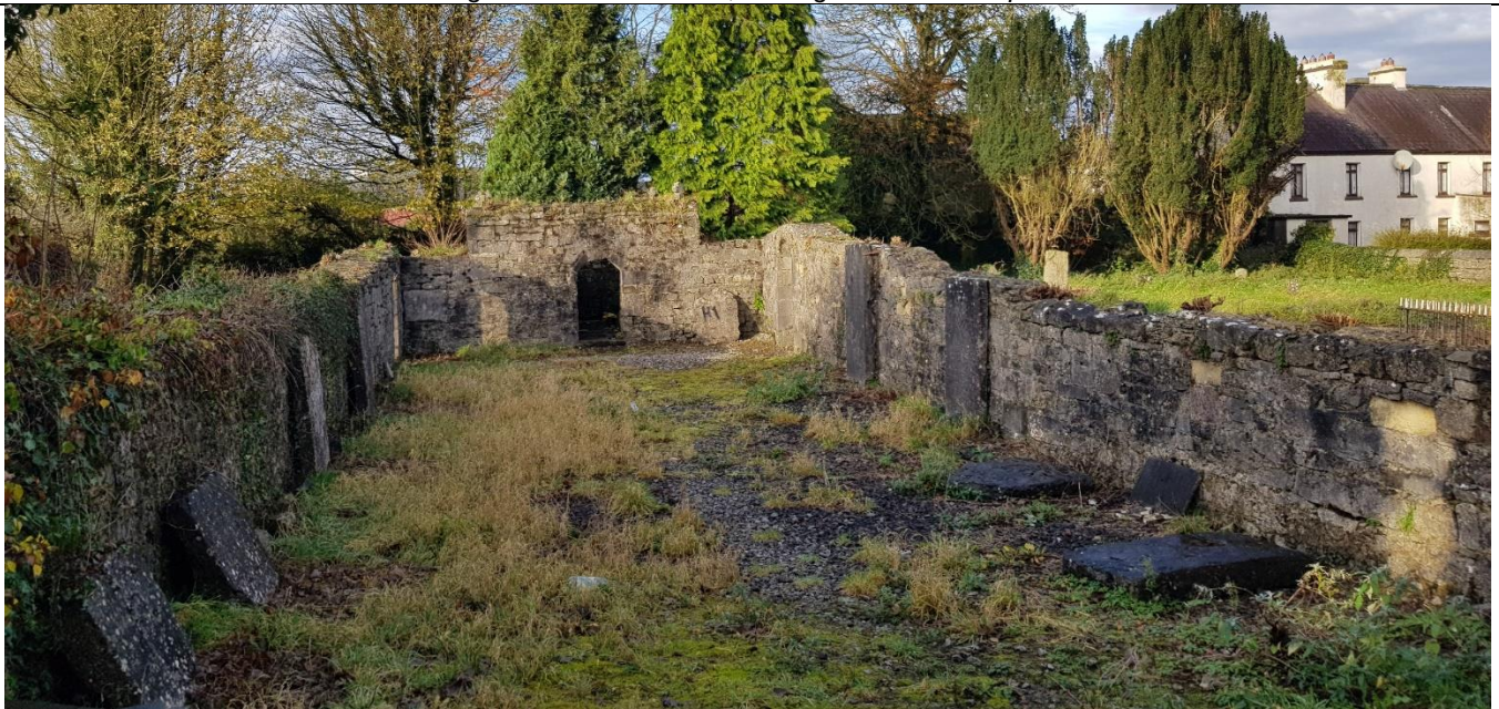
Fig. A3 Interior of nave, looking west towards tower
