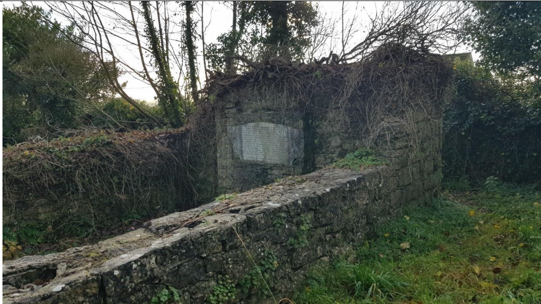
Fig. A46 West façade of chapter room
