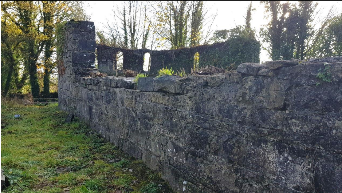
Fig. A33 North façade of nave, looking east towards apse
