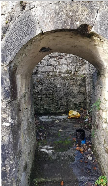
Fig. A21 Opening from nave into tower
