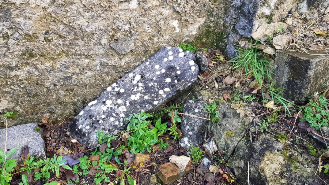
Fig. A12 Fallen headstone at north-west corner of apse
