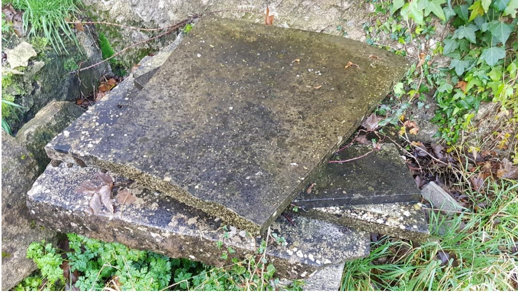
Fig. 6 Broken and displaced memorial stones within the cathedral ruin
