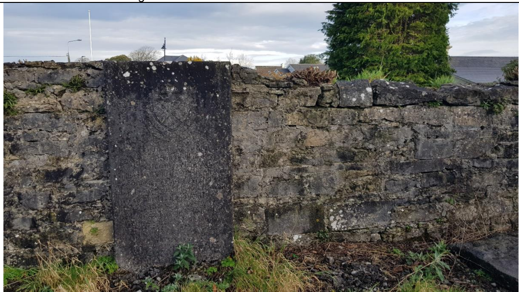
Fig. A6 Internal face of north external wall to nave
