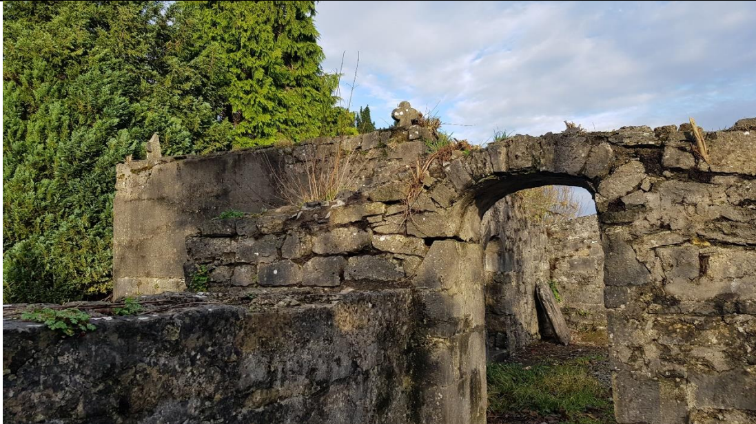
Fig. A30 North-west corner of chapter room, with opening into nave
