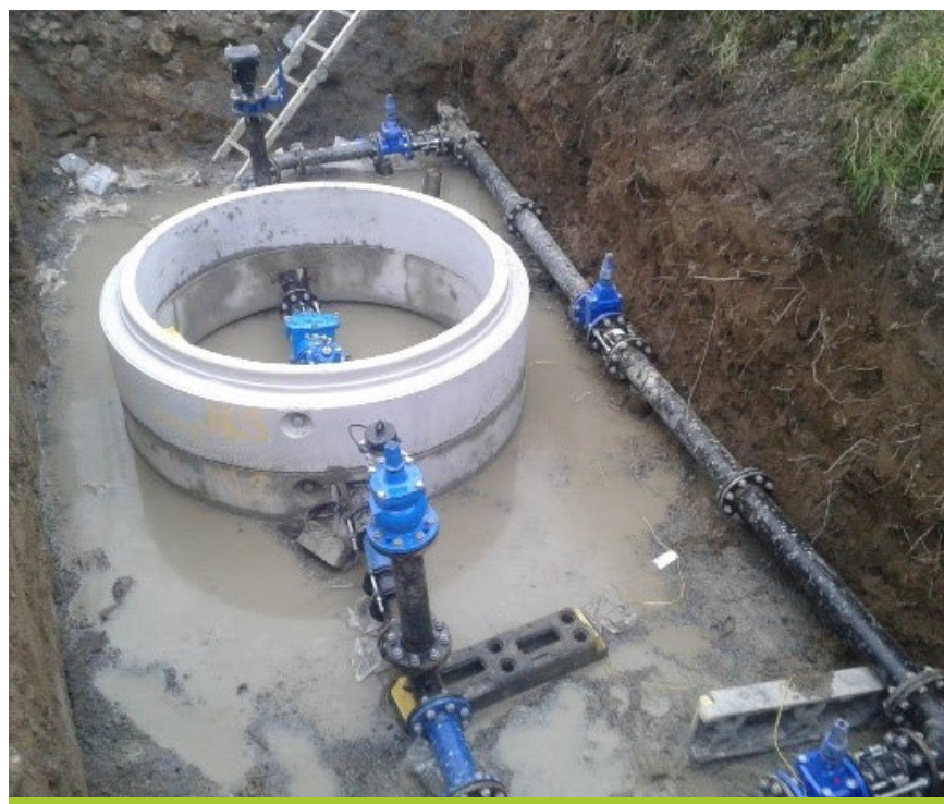
Pressure Reducing Valve and Associated Pipework at Cloonbunny District Metered Area, Ballinlough Water Supply Zone
