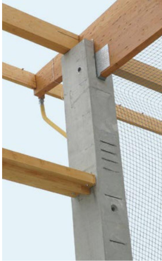
Fig. 2 Concrete post to glulam rafter connection examples
