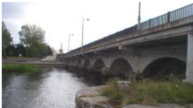
Lanesborough bridge &amp; road to hot water stretch
