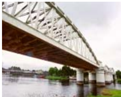
Shannon railway bridge, Athlone
