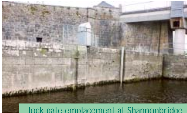
lock gate emplacement at Shannonbridge
