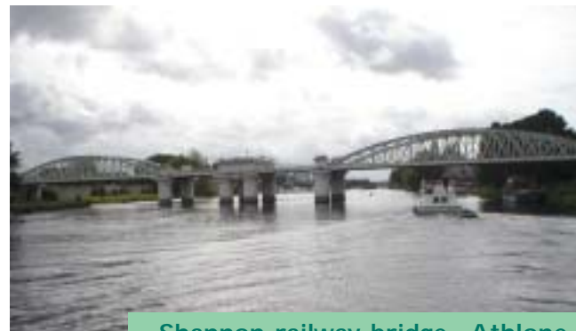
Shannon railway bridge, Athlone
