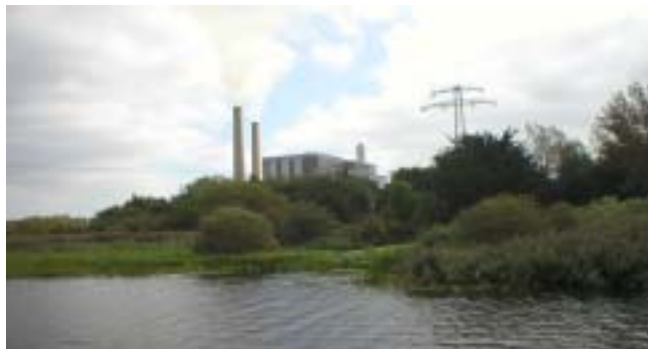
ESB power station, Lanesborough
