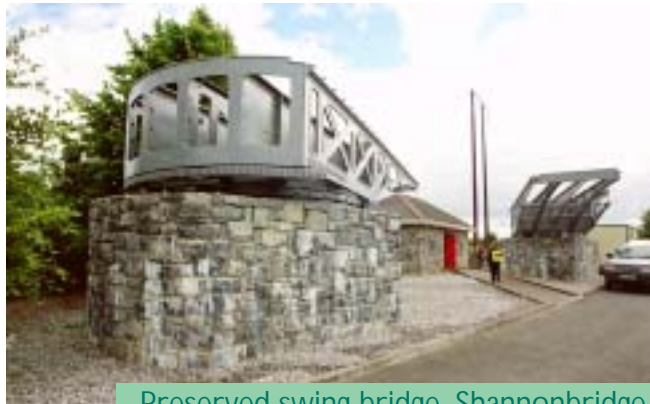
Preserved swing bridge, Shannonbridge
